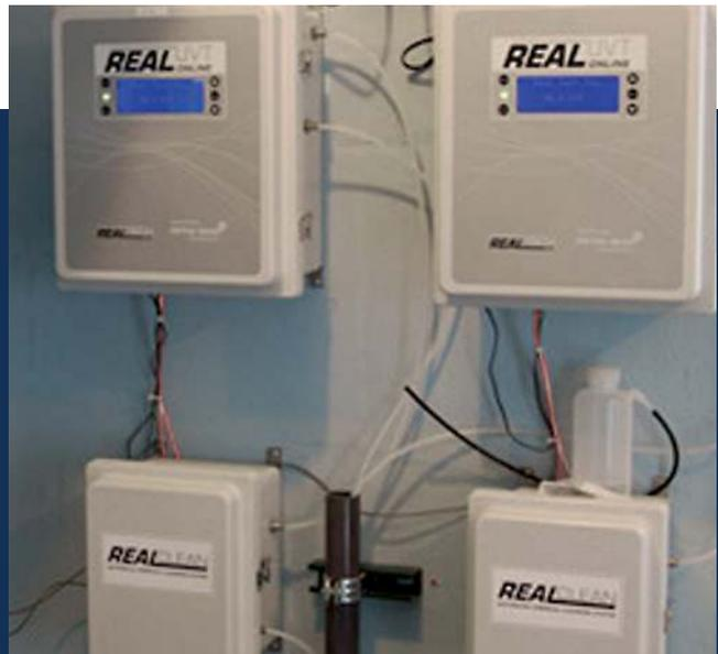
Figure 1: Real UV254 M3000 analyzers with Real Clean systems installed at MWVA WTP.
