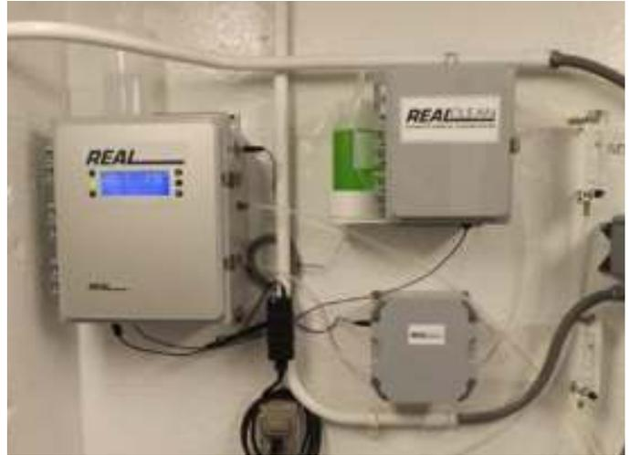
Figure 1: Ridgway WTP's Real UV254 analyzer measuring both raw and finished water with the dual feed system.
